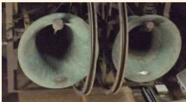
Bells No. 4 and No. 5 in the upper tier of the bellframe: these are especially tricky to ring due to movement in the frame. Photo by Robert Lewis
